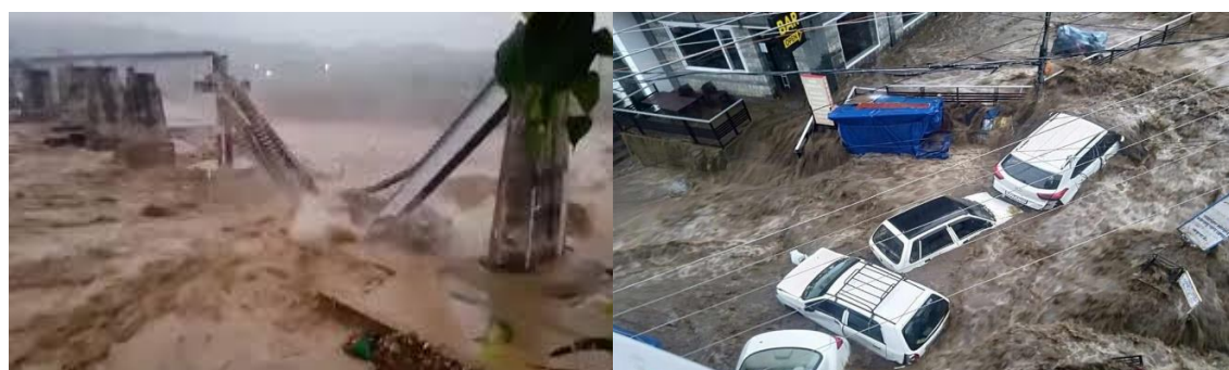
Figure 5 Collapse of Chakki bridge 2022, Figure 6. flash flood after cloud Burst in Dharamshala 2021
